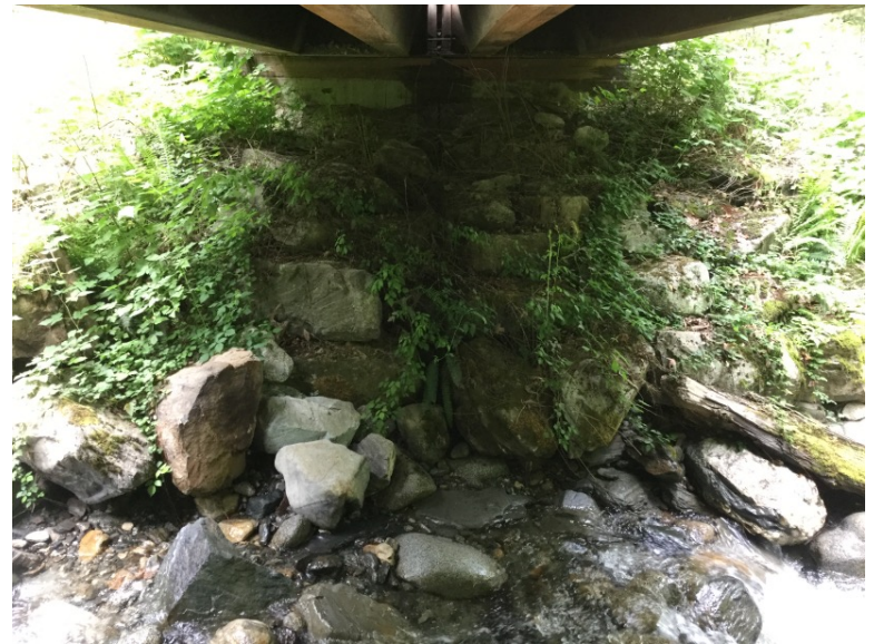
Left Bank Abutment when facing downstream
