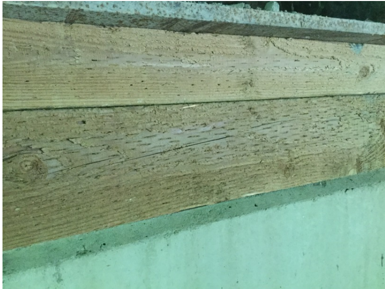
100mm thick timber on top of 150mm thick timber at both abutments
