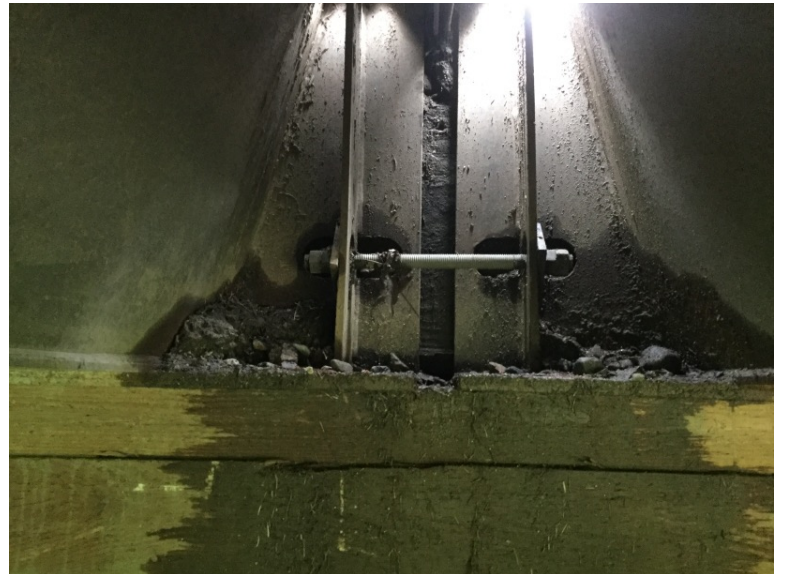
Girder connection at right bank
