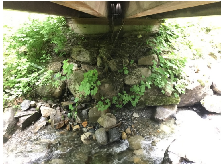
Right Bank Abutment when facing downstream
